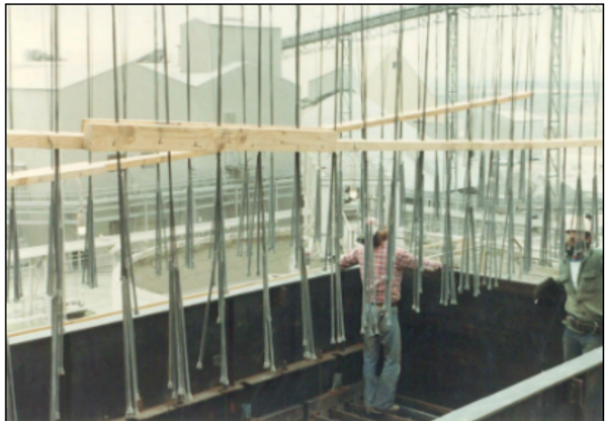
Installing precipitator wires (discharge electrodes)
