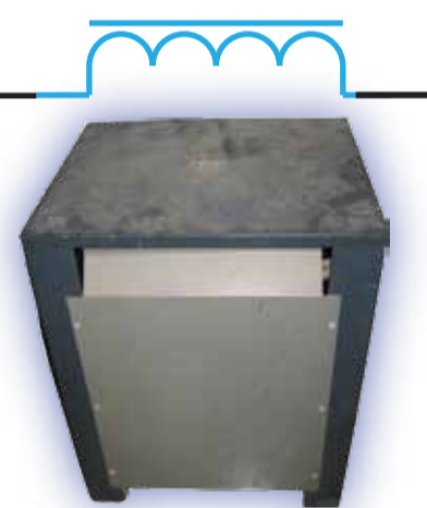
CURRENT LIMITING REACTOR (CLR)
