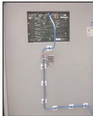
Cabinet interior with more compact logic and interface boards and streamlined connections
